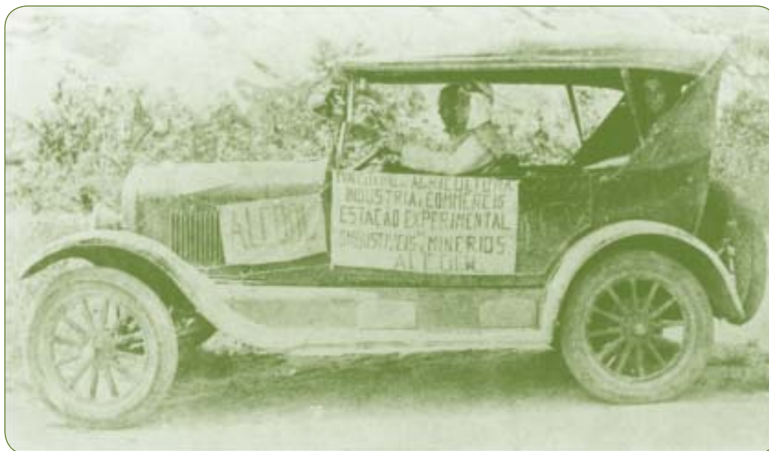
Ford vehicle adapted by INT in 1925 for demonstrations of the use of bioethanol as fuel.
